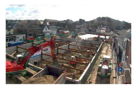
Figure 2. Construction of an infiltration basin in the heart of Egmond aan Zee.
